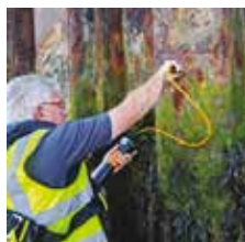
Marine Asset Inspection
